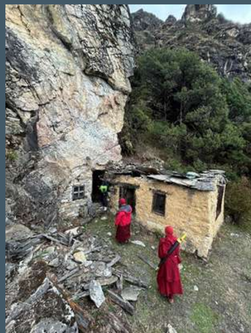
THE EARTHQUAKE DAMAGED EXTENSION TO A RETREAT CAVE, PHORTSE
